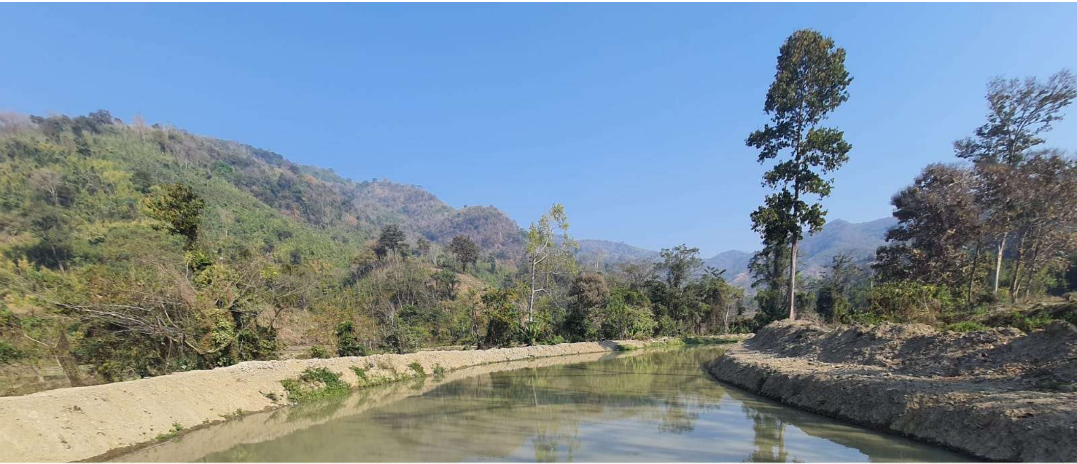
New Pond Construction (2020-2021) Name of Beneficiary : C.Sado of Kiasi
